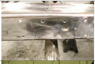
You should be left with only your trace marks for where to cut for the c-notch
