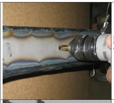
Drill the frame through the existing 3/8" hole in the boxing plates to make the locating point for the cross member.
