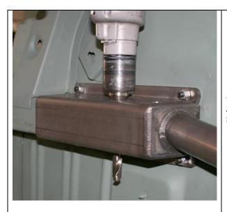
Afterward you can run the drill through both holes to insure the bolts will go through clean. Hang onto the drill; it will want to grab the frame sheet metal.
