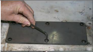
Remove the one 5/16 locating bolt, place the inside reinforcing plate over the six drilled holes. Using the six button head bolts, washers and nuts per side, tighten the plate down against the floor with heads of the bolts and washers on top and the nuts on the bottom against the channel flange.
